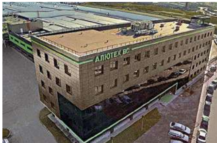
Alutech Doors Systems LLC
